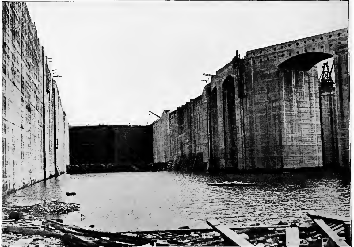
WALL OF GATUN LOCK SHOWING ARCHED CONSTRUCTION
